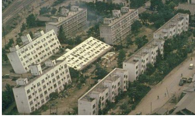
Figure 2-11: Example of Bearing Capacity Failure During the 1964 Niigata, Japan Earthquake (Photo from quakeinfo.ucsd.edu/ )
